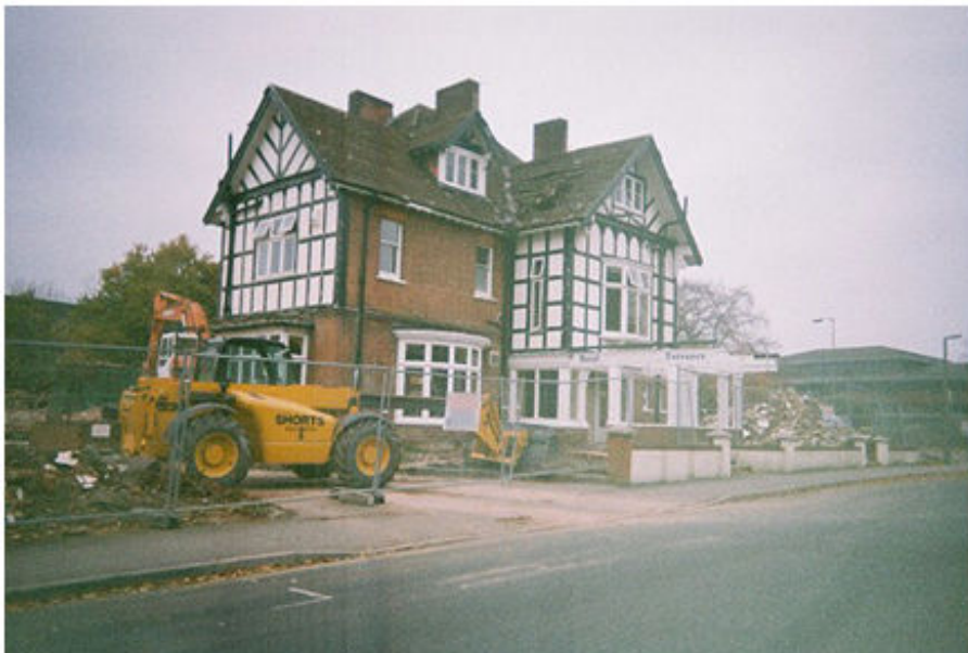
Figure 15. Old building, soon to be demolished
