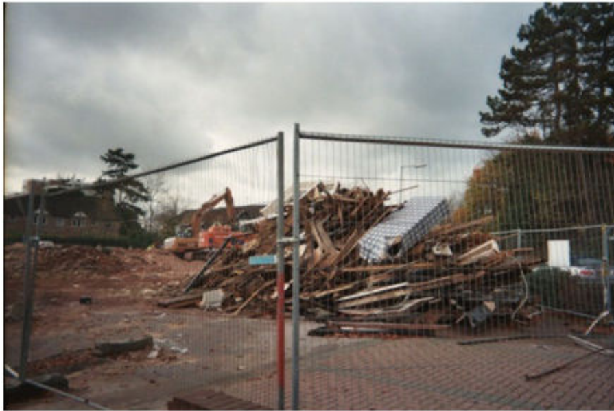
Figure 16. All that is left after the demolition
